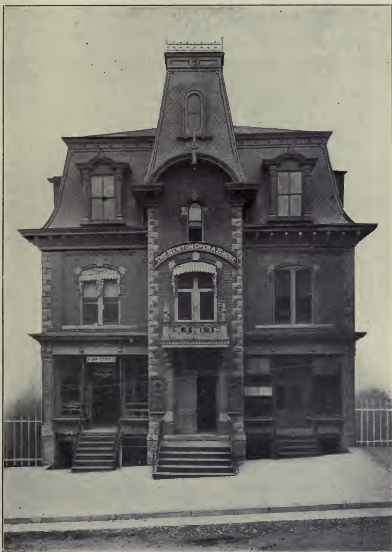
DENNIS LIBRARY BUILDING. Newton, Sussex County, New Jersey.
